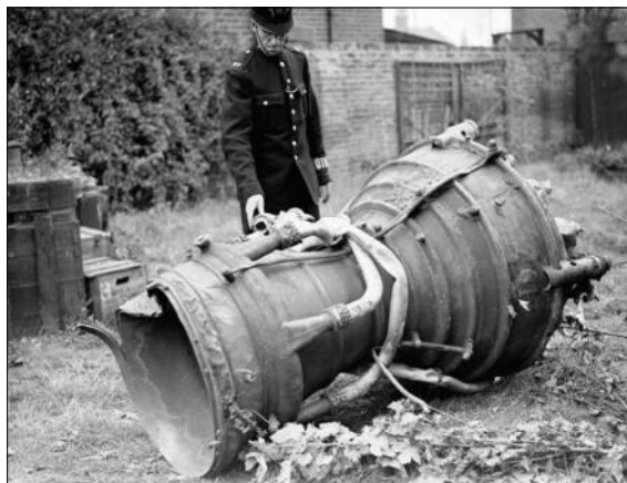
A police officer examines the remains of a V2 that hit London in September 1944.
